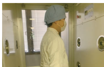
Air shower before entering the SPF area
